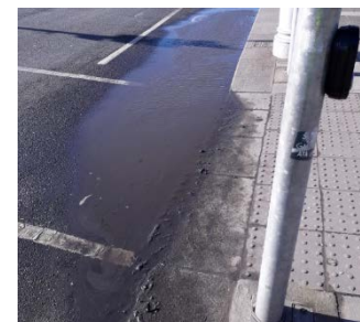
Figure 20 Example of existing drainage issues at existing crossing on Custom House Quay
